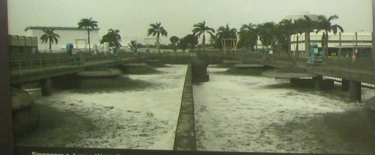
Singapore • Jurong Water Reclamation Plant MBR (Singapore's largest MBR plant) Capacity: 68,000m 3 /day. Completed: 2011
